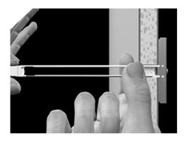
B Hold ends of straps between thumb and forefinger and pull toward you until channel rests flush behind wall. Slide plastic cap along straps with either hand with flange of cap is flush with wall.
